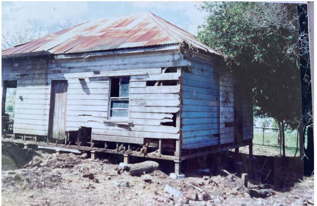
Figure 125: View of southwest corner of the building showing the enclosed ends of the verandah already demolished.
