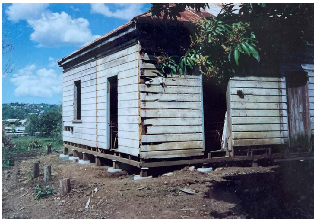
Figure 127: View of the northwest corner of the building showing remnant verandah post footings. Source: Photo supplied by Craig and Jane Murray.
