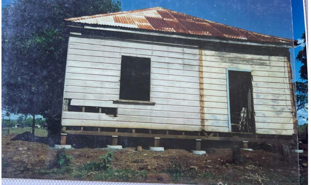
Figure 124: View of the north elevation showing the enclosed ends of the verandah already demolished.
